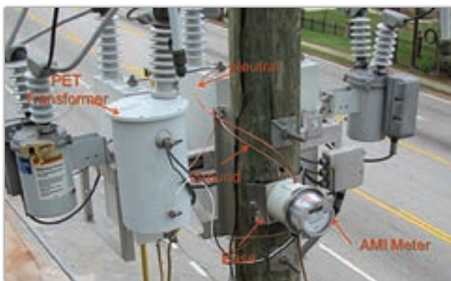
Installation of the Advanced Meter Capacitor Bank Health Monitor
